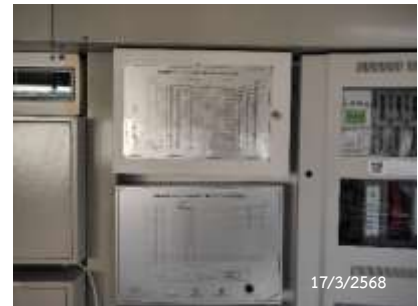
Graphic Annunciator Fire Alarm System
