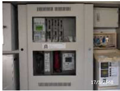
Fire Alarm Control Panel
